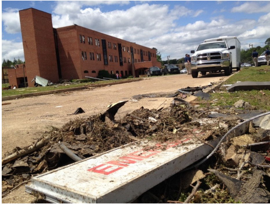
Figure 2. Wayne General Hospital after 2014 Tornado, Photo Courtesy of Aircare
